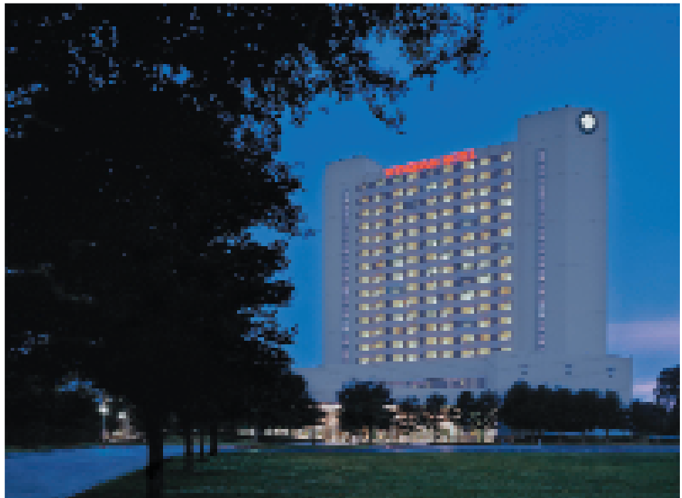
Texas Fire Protection Systems overhauled The Wyndham Arlington's primary fire safety equipment in less than 2 weeks to ensure that all rooms would be ready for the spring influx of Texas Ranger fans.
