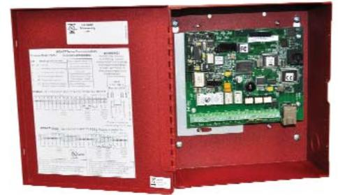
If using the IP Communicator with the 5104 digital communicator, order the IPDACT-2 and the HP300ULX.
