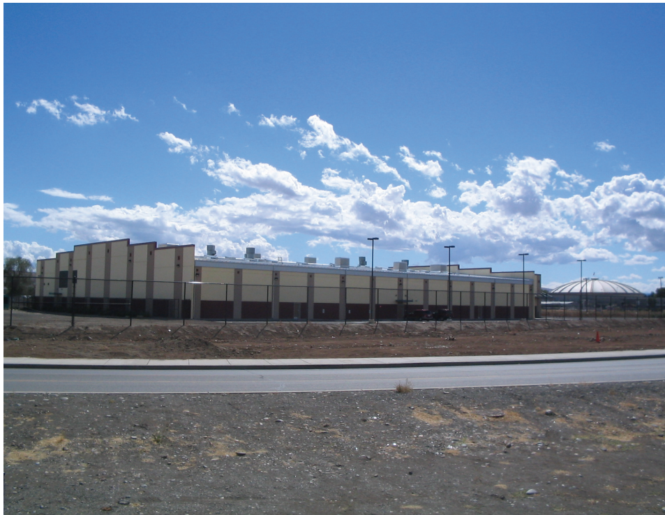
Yakima Valley Justice Center protected by IFP-1000 Panel.
